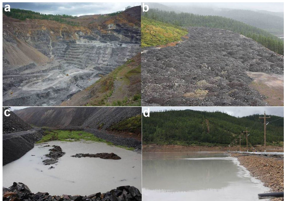
Fig. 2 a Quarry of the Anfishinsky ore deposit; b overburden dumps; c settlement pond; d tailings dump
